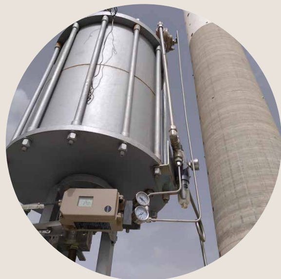
Fig. 9. Molten salt pump recirculation with detail of the concentric tower thermosolar power plant
